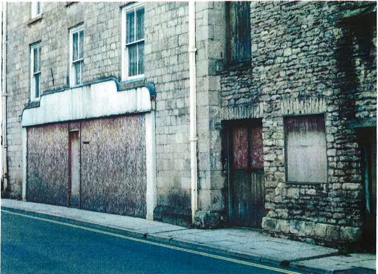
COMMERCIAL DETERIORATION OF OXFORD STREET NOVEMBER 2011
